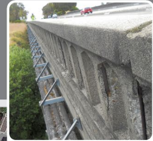
Telecommunications on North Side of Existing Bridge Utilities must be protected in place or relocated (temporary or permanent).
