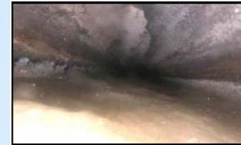
MH 2 to Vault 1 at 0 feet - Corrosion and grease, typical throughout project area.
