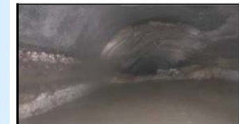
Vault 8 to Vault 7 at 270 feet - Grease/blockage in flow and corrosion/spalling from 9 to 3 o'clock.
