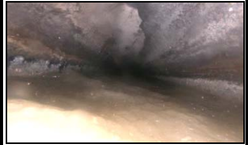
MH 2 to Vault 1 at 0 feet - Corrosion and grease, typical throughout project area.
