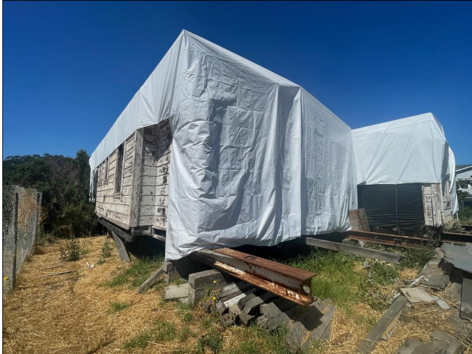
Corner of subject structure supported above steel I-beams.
