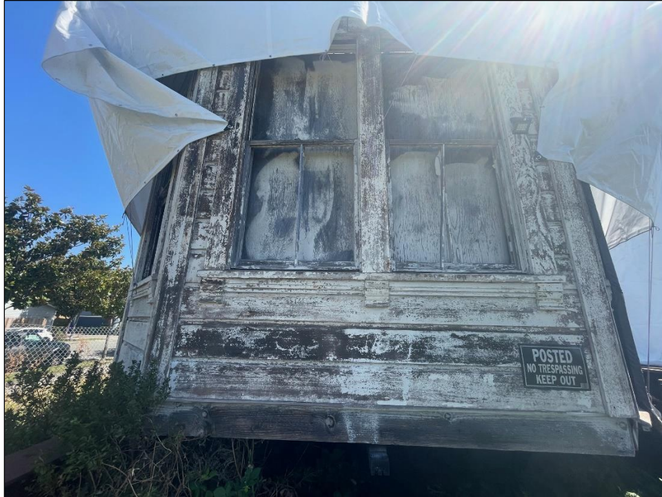
Angled bay window partially exposed from the temporary tarp.
