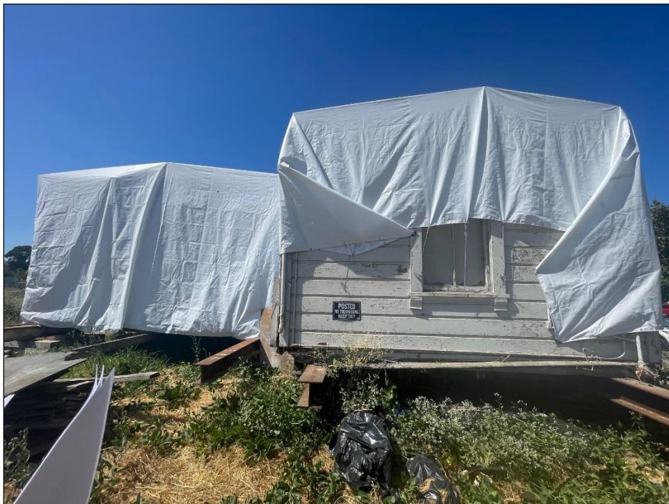
Side of subject structure with one window partially exposed.
