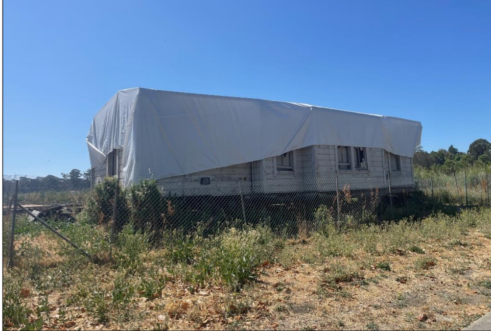
Overall length of subject structure with temporary tarp.
