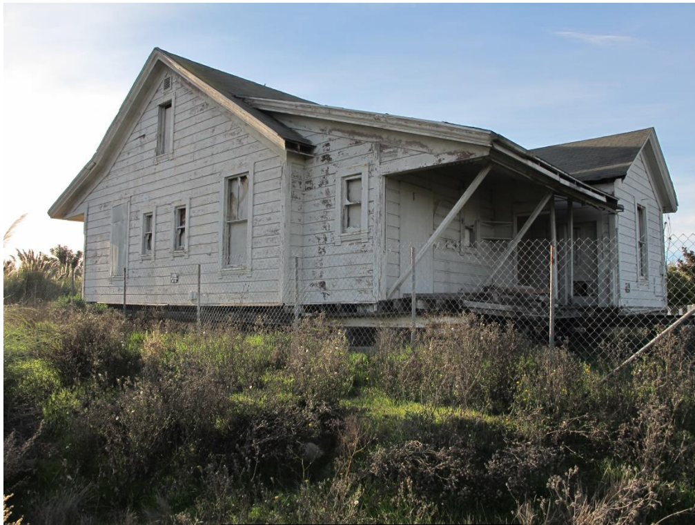
Rear Elevation, November 2017
