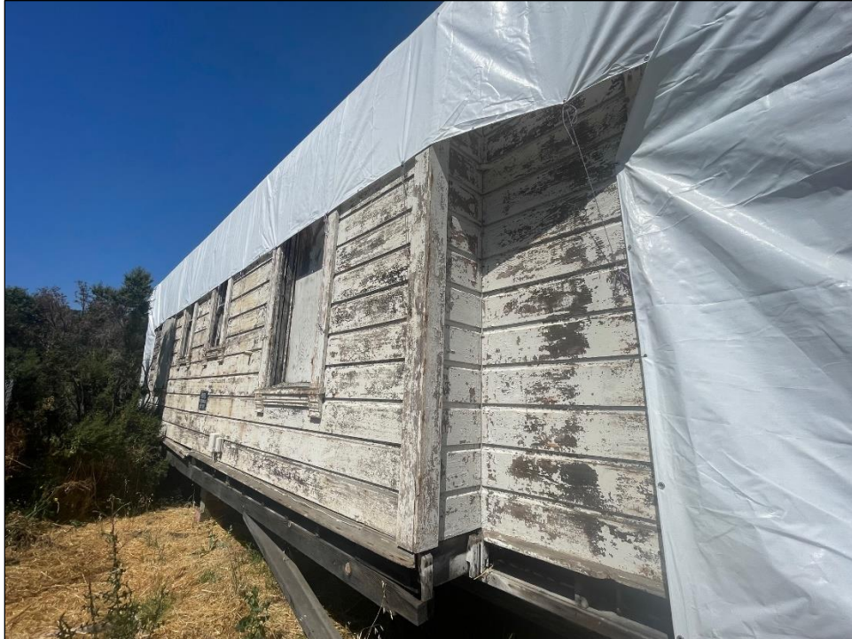
Side of subject structure with three windows partially exposed.
