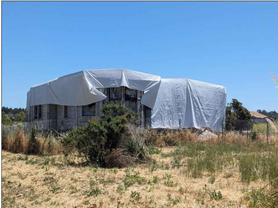
Subject structure at current temporary location (City's Corporation Yard) with roof removed and with temporary tarp. Prior to August 2024.
