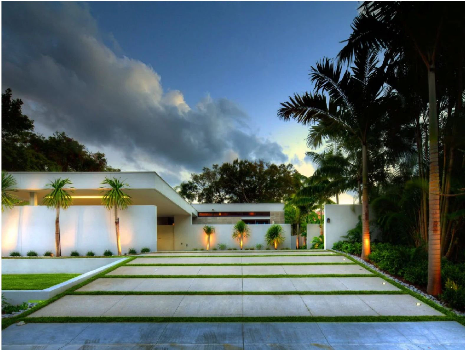
Concrete Paver Driveway w/ Grass Smooth Stucco Site Walls, Cream
