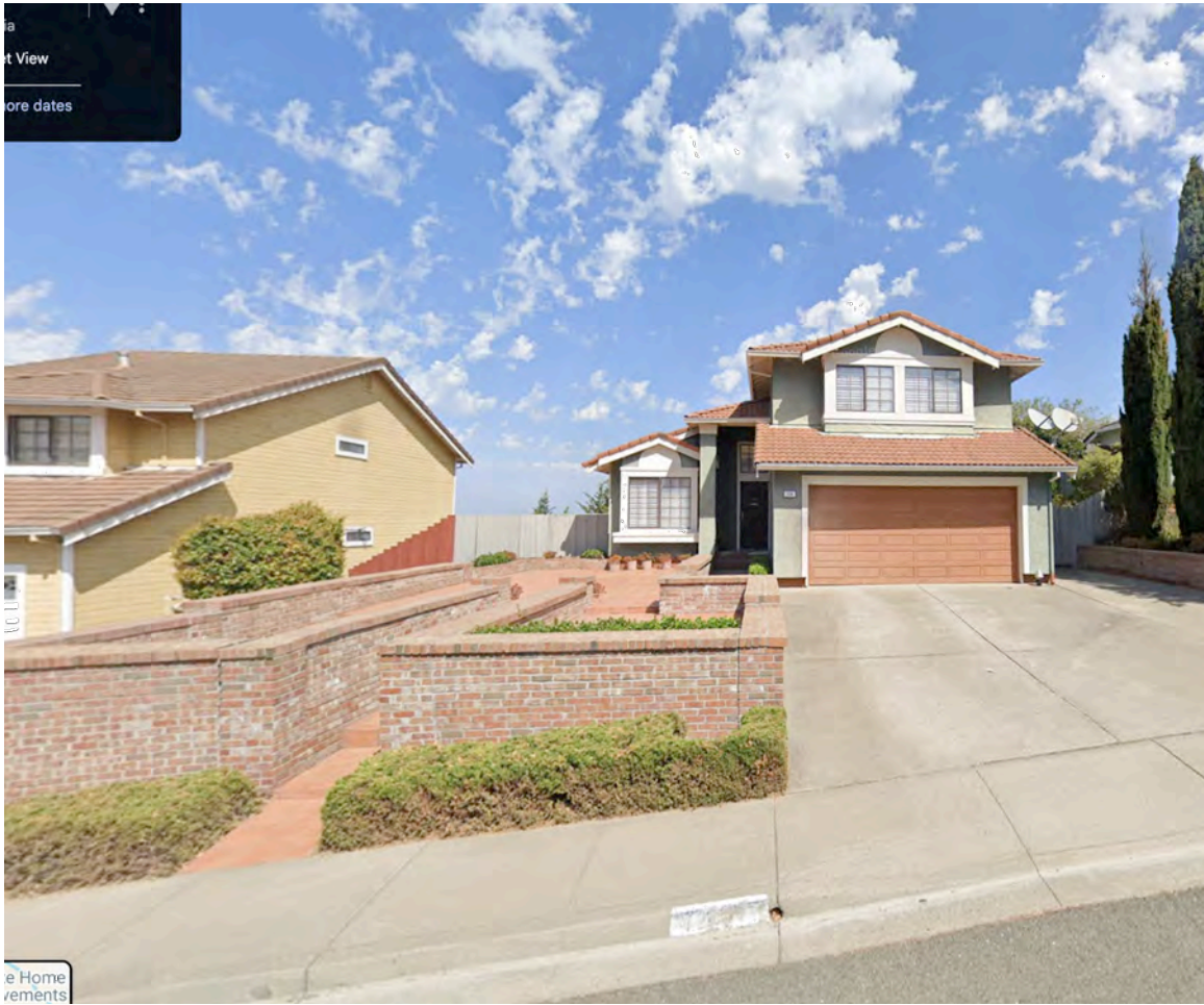
Front Yard Landscape Walls & Steps
