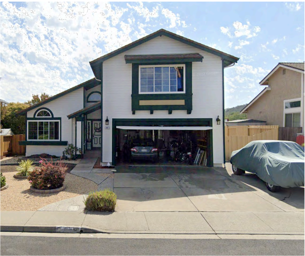
2-Story Gable Front Massing Contrasting Light Walls & Dark Accent Color
