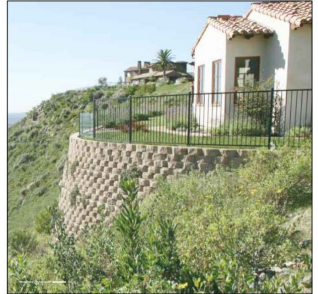
TYPICAL GRAVITY BLOCK WALL (MSE WALL)
