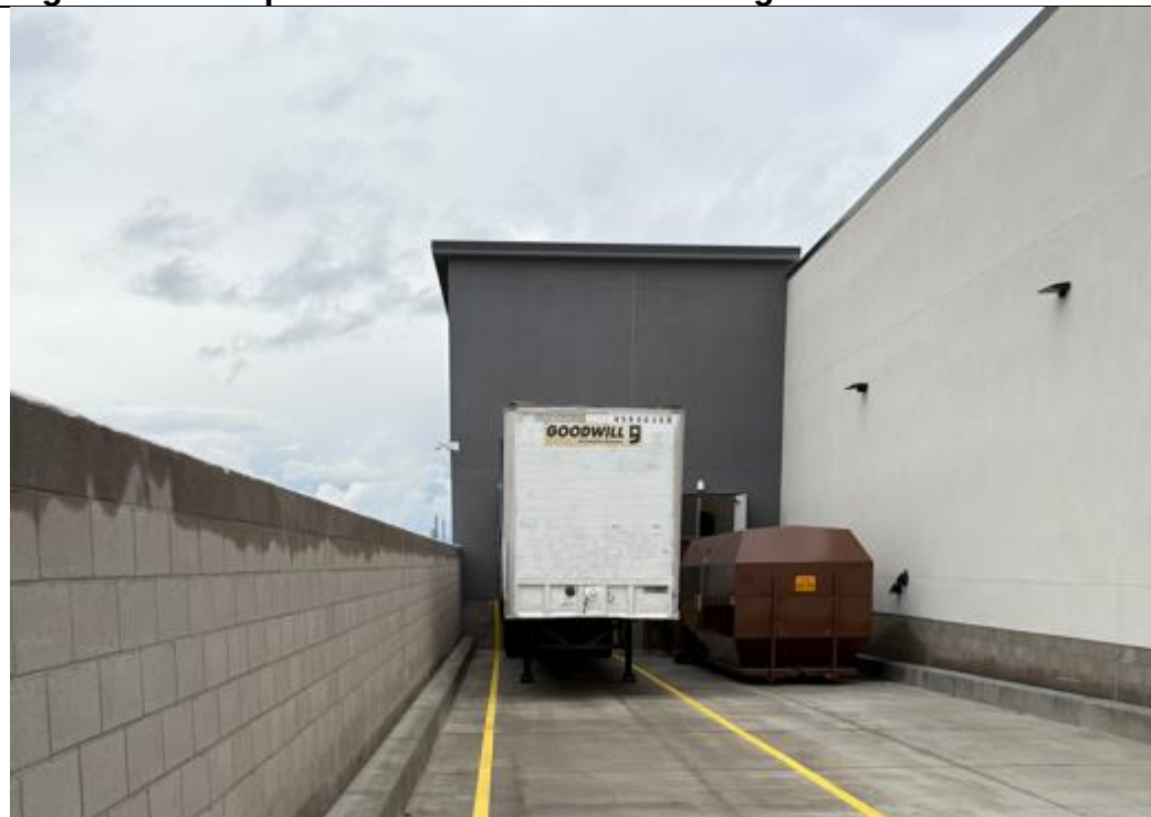
Figure 6: Example Photo of Goodwill Loading Dock Area
