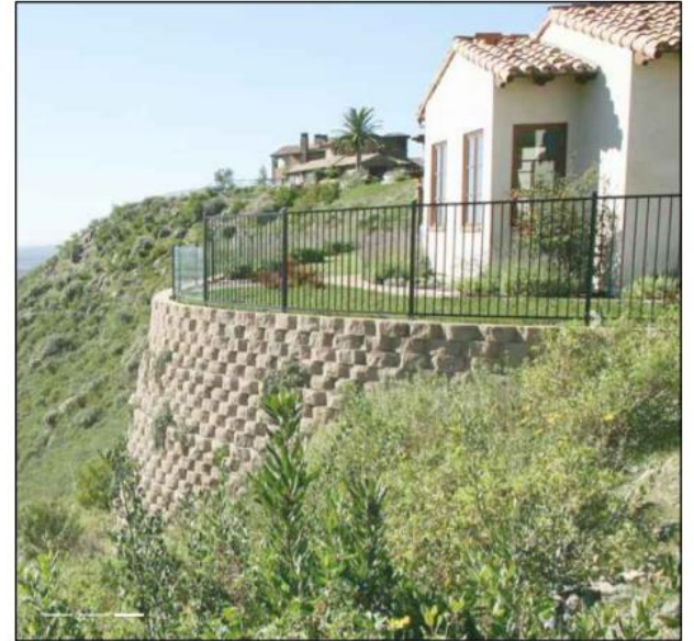
TYPICAL GRAVITY BLOCK WALL (MSE WALL)
