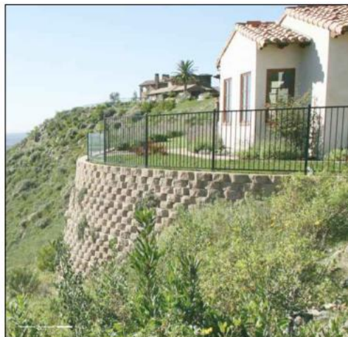
Figure 11: Typical Gravity Block Wall
